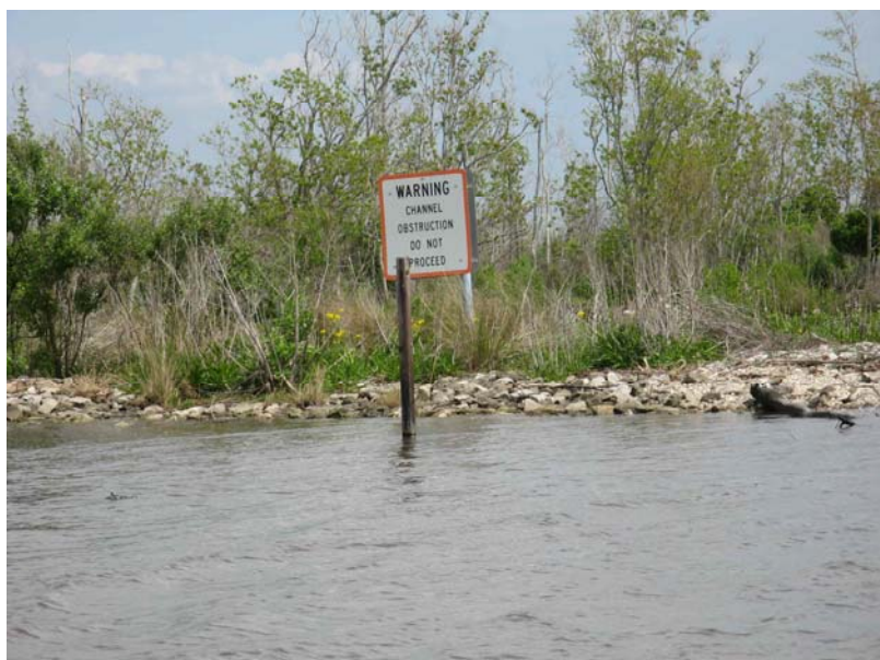
Photo 7 Low area in Structure #17
