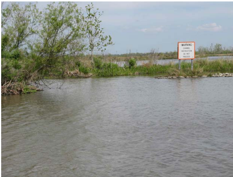
Photo 3 Breach on west side of Structure #14
